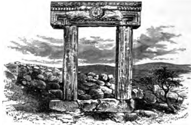
DOOR-POSTS AND LINTEL OF RUINED SYNAGOGUE.
